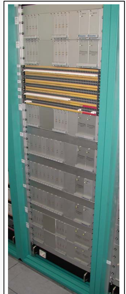
Fig.3 19"/3RU frames for AD/DA converters DUAL and digital distribution amplifiers with two power supplies
